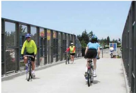
Figure AE-3.1: Bicycle and Pedestrian Bridge. Photo by CH2M Hill.
