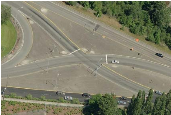
Figure MR-2.3: A paved non-accessible median (image from Bing Maps).
