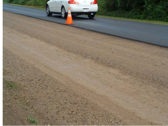
MR-2.15: Finished FDR material before overlay (photo from Grace Pacific, Inc.).
