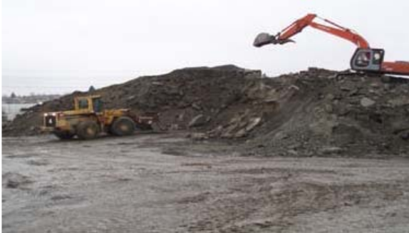
Figure PR-6.1: Typical pile of roadway construction waste. (Bremner and City of Vancouver 2006)
