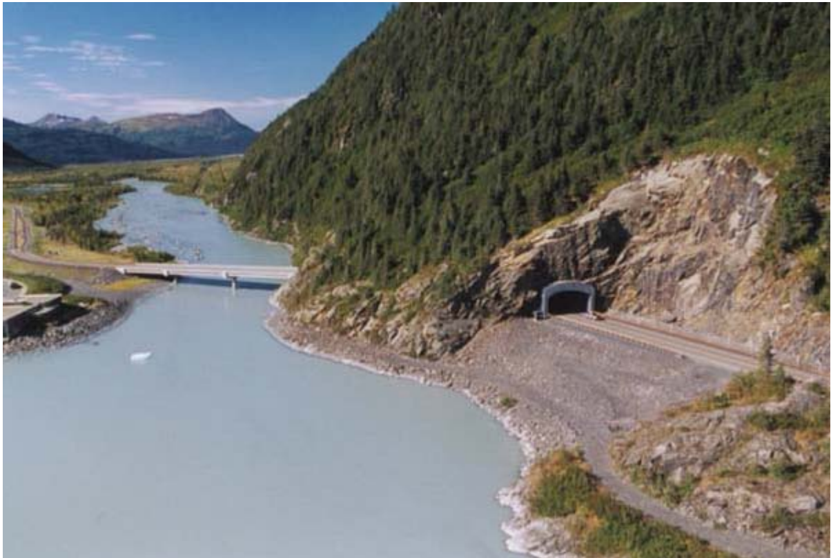
Figure AE-3.4: Whittier Access project. Photo by CH2M Hill.
