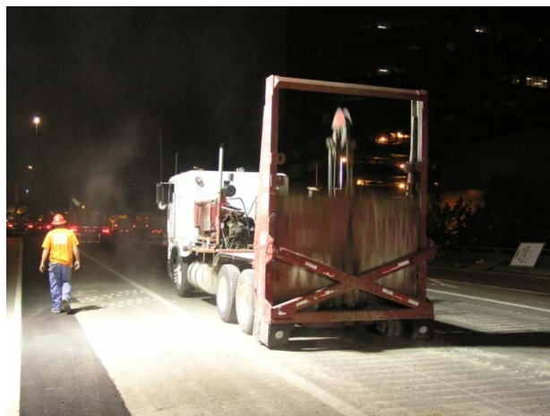
Figure MR-2.16: Guillotine breaker used for crack-and-seat.
