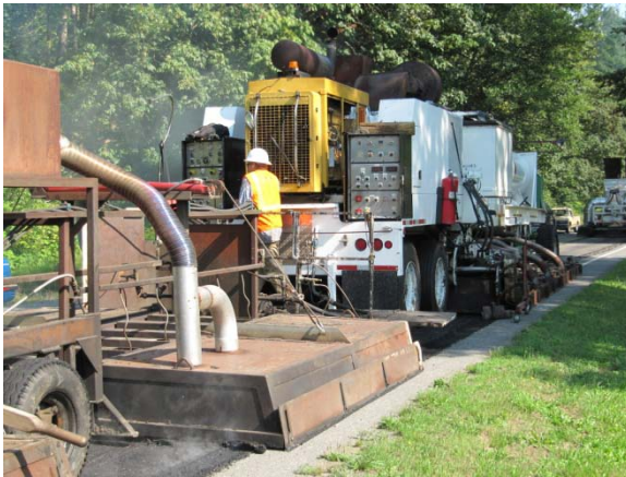
Figure MR-2.11: HIR heating equipment.
