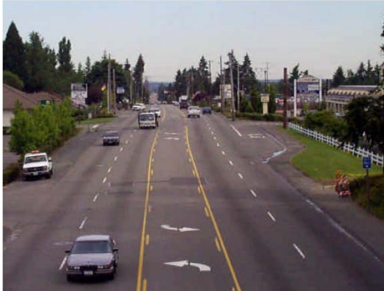
Figure AE-6.4: Bridgeport Way Before Construction. (Context Sensitive Solutions, 2005)
