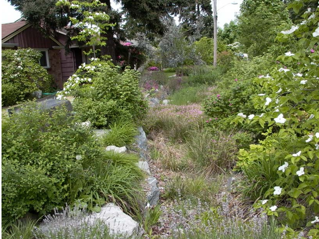
Figure EW-3.1: A well-established vegetated swale (“bioswale”) that uses compost amended soil and no flow control devices or structures. Residential street to right. Seattle, WA. (Photo by J. Anderson)
