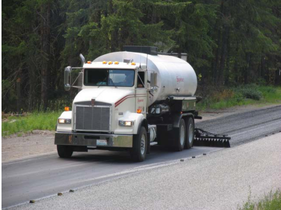
Figure MR-2.7: Chip seal asphalt emulsion application.
