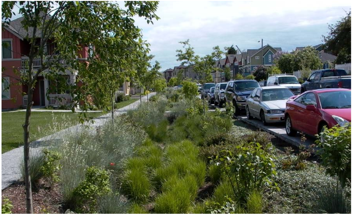
Figure PR-8.1: Three LID techniques are featured in this photo taken at High Point Subdivision in Seattle, WA. The grassy area (far left) is actually turf placed over a large infiltration basin. A bioswale (center) is featured, and still in early growth. Also, the sidewalk (left) and the street (right) are paved with permeable concrete. (Photo by J. Anderson)
