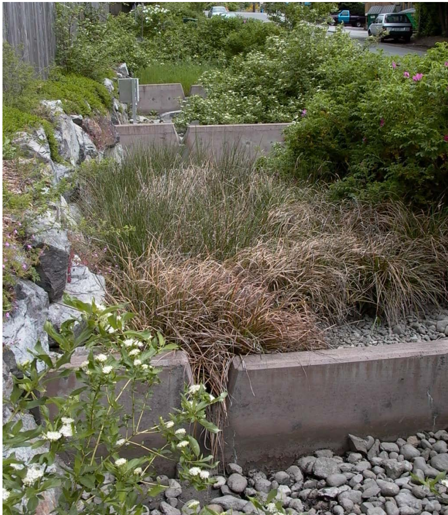
Figure EW-2.1: A bioswale with flow control weirs. (Photo by J. Anderson)
