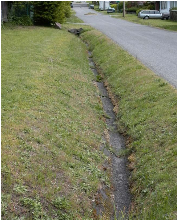
Figure PR-8.3: A conventional asphalt lined channel near SEA Street. (Photo by J. Anderson)
