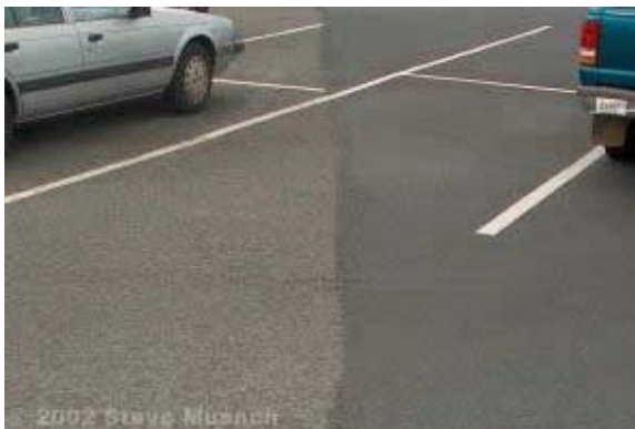
Figure MR-2.5: No fog seal (left), fog seal (right).
