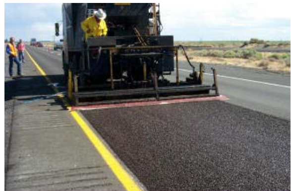
Figure MR-2.6: Microsurfacing (from the Washington State Department of Transportation).
