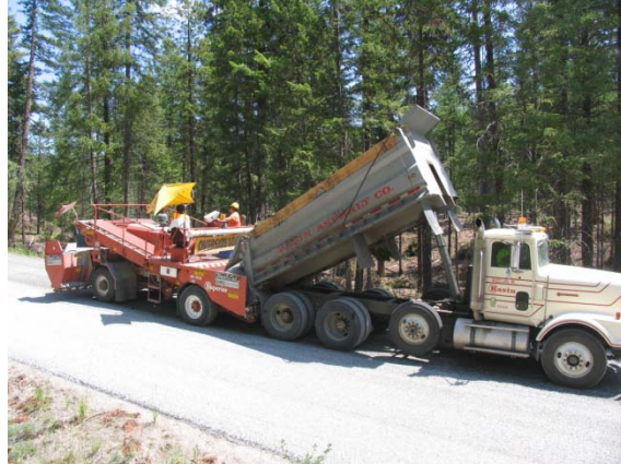
Figure MR-2.8: Chip seal aggregate application.
