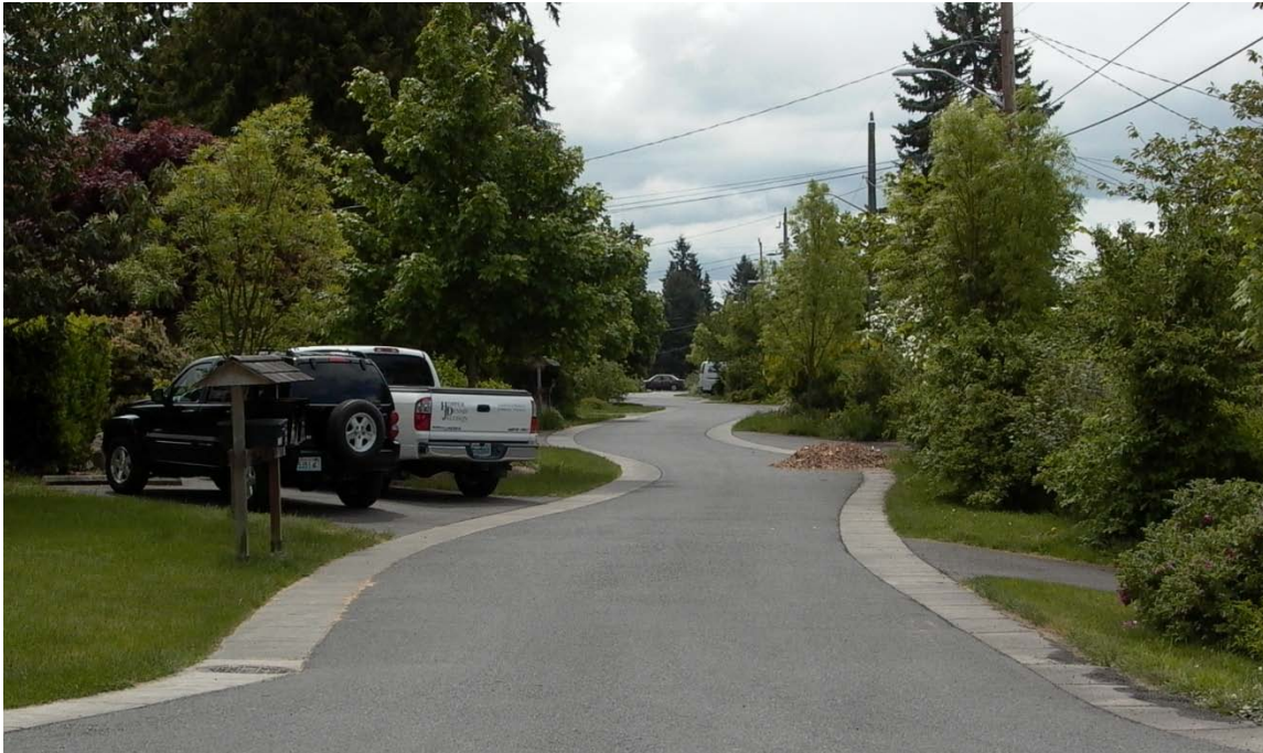
Figure PR-8.2: This street was designed to be narrower in order to produce a traffic calming effect for this residential area. (Photo by J. Anderson)
