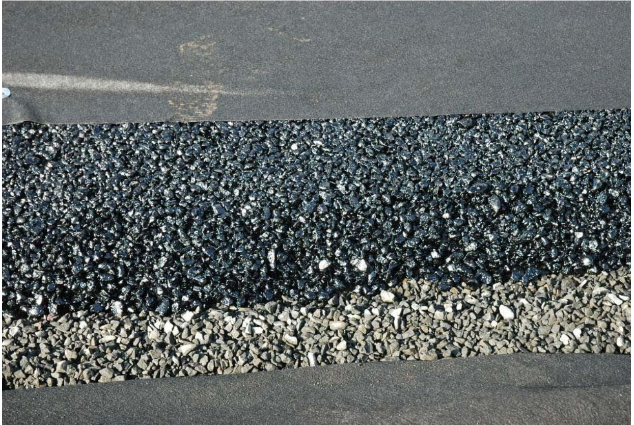
Figure PT-2.1: The appearance of porous asphalt is much the same as non-porous asphalt. The porous asphalt is placed over course of porous aggregate beneath a temporary geotextile fabric, which is to prevent clogging issues during construction. (Photo by K. Hansen, National Asphalt Pavement Alliance)
