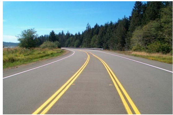
Figure MR-2.4: A paved accessible median on US 101 in Washington State.
