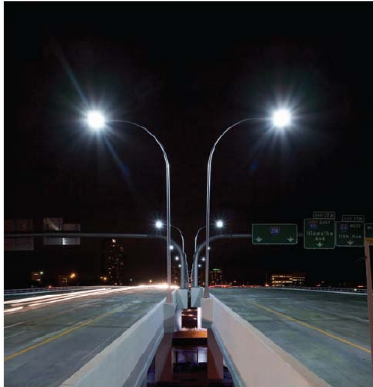
Figure MR-6.2: Lit LED luminaires at night on I-35. Photo by Figg Engineering Group. ( http://www.ledwaystreetlights.com/Benefits/pdf/case-study/ledway-I-35W-CaseStudy.pdf )
