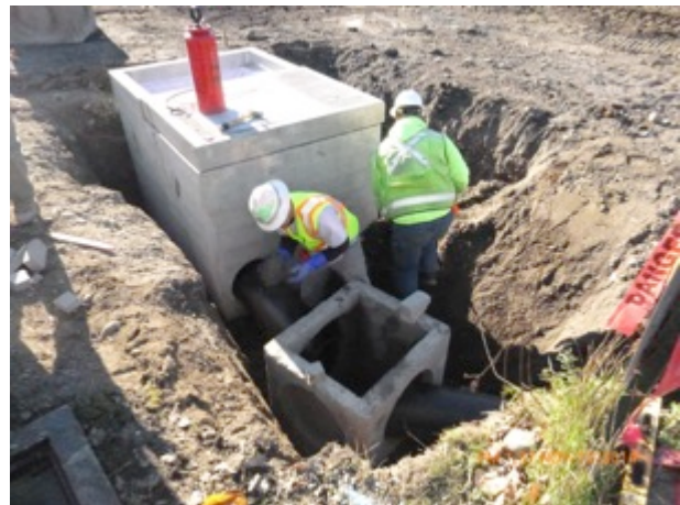
The bridge has its own biofiltration in tiny wetlands at the edges to treat and manage runoff - bioclean modular wetlands
