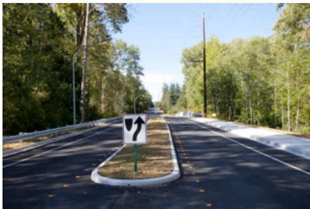
Total area of warm mix asphalt: 5.590 square yards
