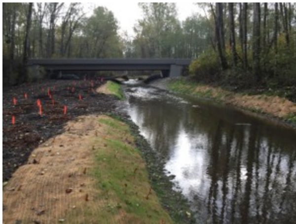
Habitat restoration was a point of pride for this bridge project.
