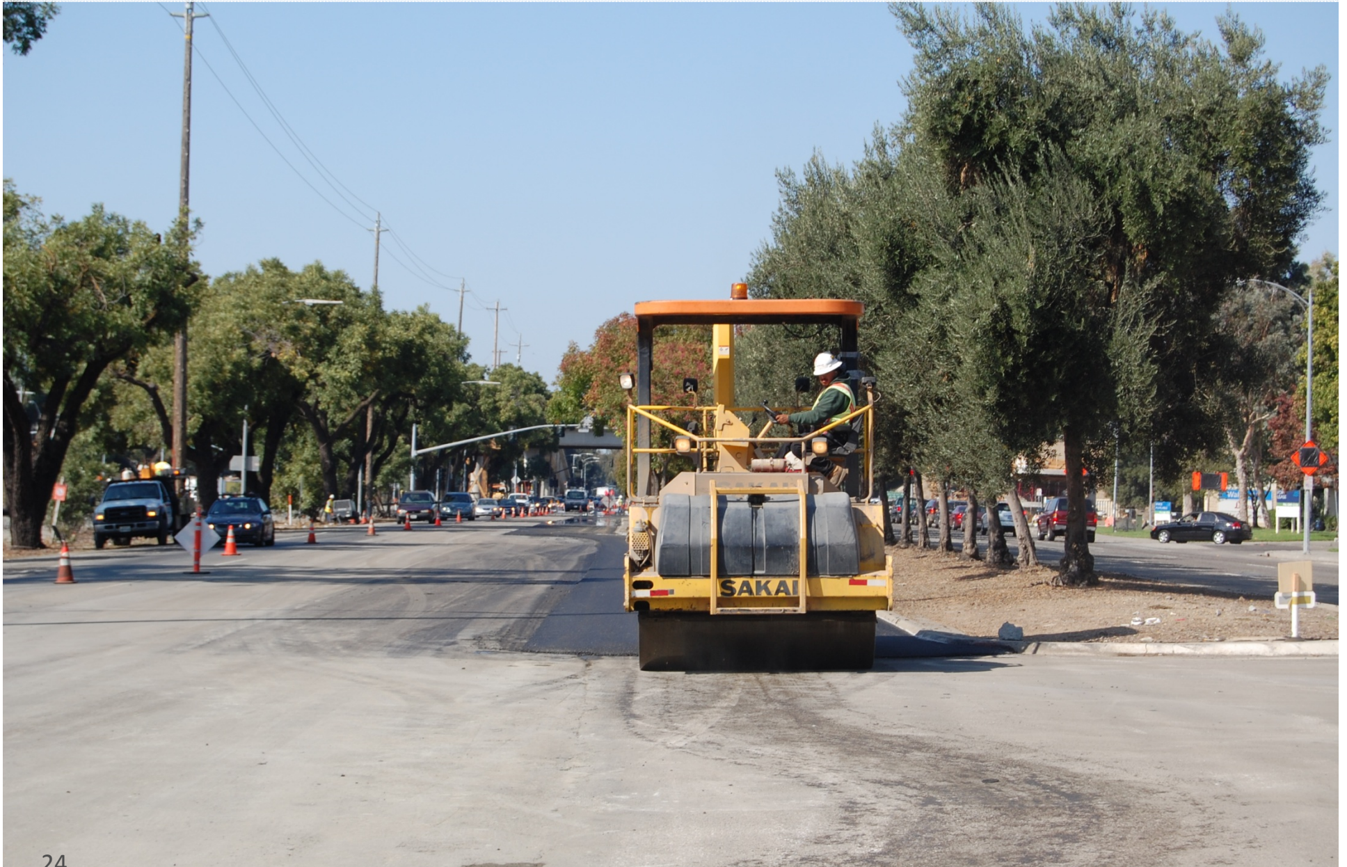
Placing the HMA wearing course over cold-in-place recycled base. Monterey Road Reconstruction, San Jose, CA
