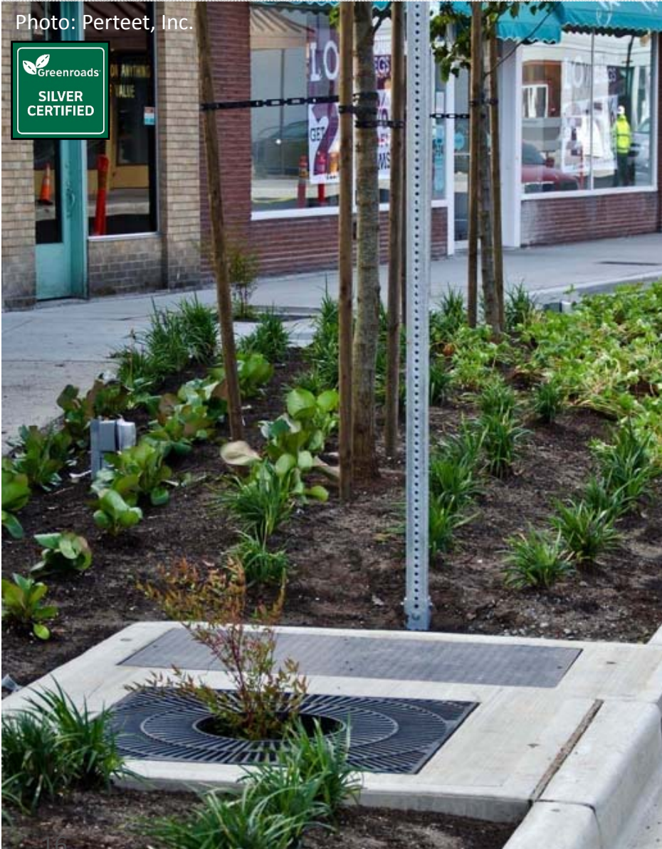
Filterra stormwater unit (left) in Oak Harbor, WA and pervious concrete sidewalk (right) in Bellingham, WA
