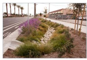
The new 2,600 foot bioswale runs between the north and south lanes. The unusually flat area created a challenging condition for managing surface runoff.
