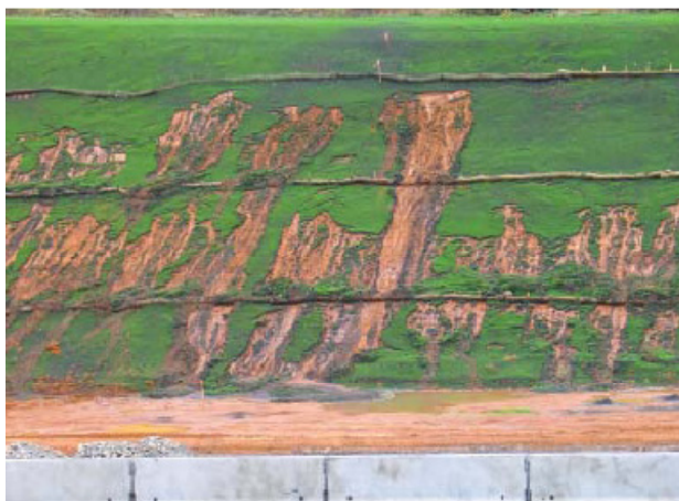
Figure EW-5.1: A failing revegetation effort on a steep slope that did not use a native revegetation approach (from Steinfeld et al. 2007a).
