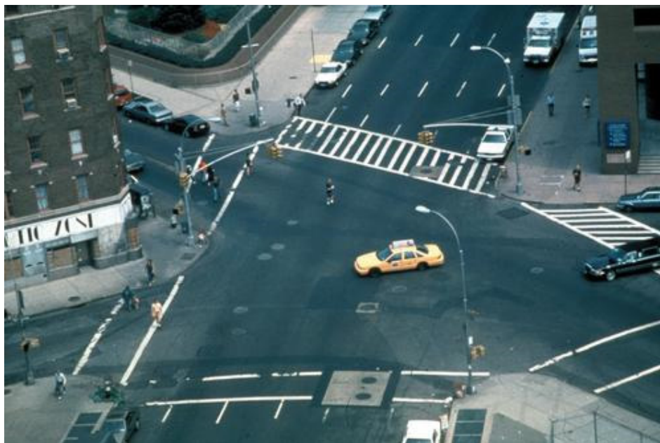
Figure AE-5.1: Mulry Square Before Construction (Context Sensitive Solutions, 2005)
